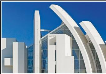
The Jubilee Church completed in 2003, is a flagship when it comes to the use of nanotechnology in construction . Nanostructured TiO<sub>2</sub> (titanium oxide) particles theoretically will keep the concrete white forever, even in smoggy Rome. The titanium oxide actually eats carbon. We use titanium oxide in the organite pendants to add some carbon eating benefits. See: <http://nextbigfuture.com> (**temple of nanoscience**)
